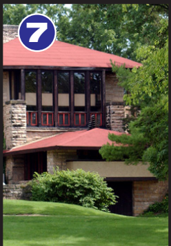
7 TALIESIN AND VISITOR CENTER
