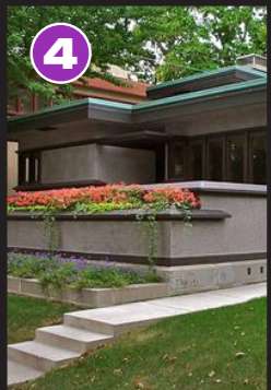
4 BURNHAM American System Built Homes
