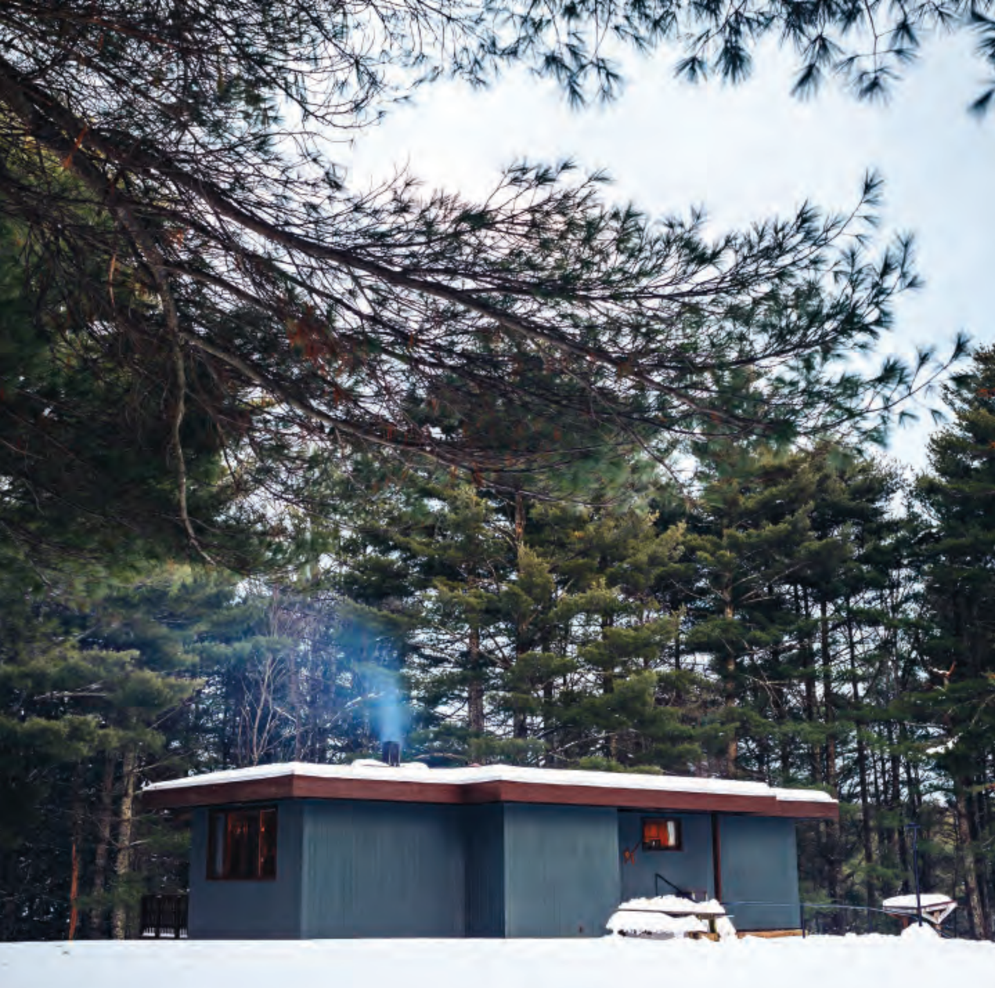
PIPESTEM RESORT STATE PARK
